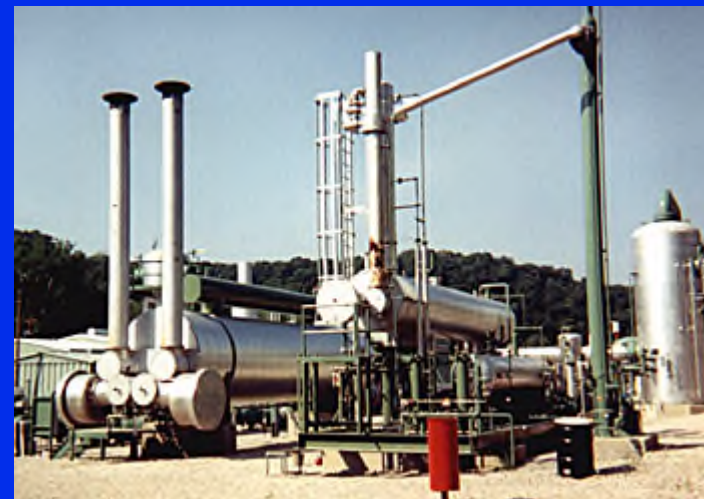
Glycol Dehydrator Unit Source: GasTech
