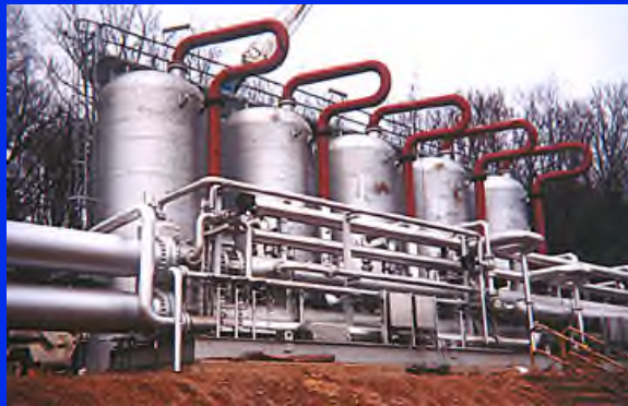
Desiccant Dehydrator Unit Source: GasTech
