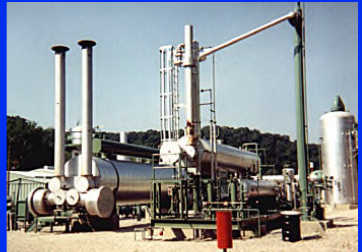
Glycol Dehydrator Unit Source: GasTech
