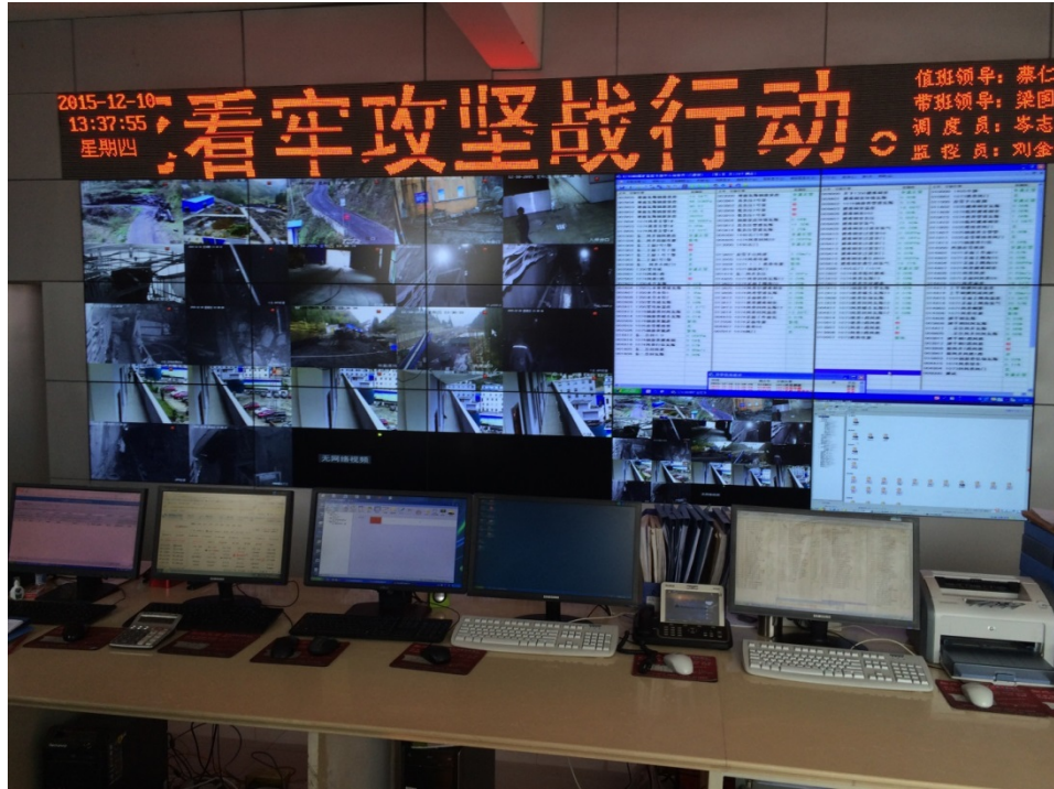
Figure 2-4: Liulong Mine State-of-the Art Control and Monitoring Room
