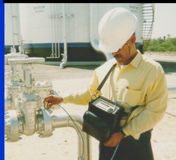
Acoustic Leak Detection
