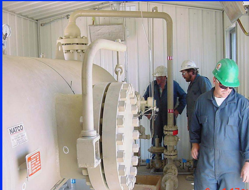
Portable Three Phase Separator, Source: BP
