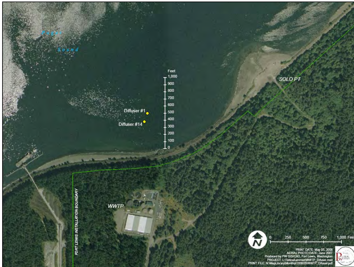
Figure 2. Facility and Outfall Aerial View
