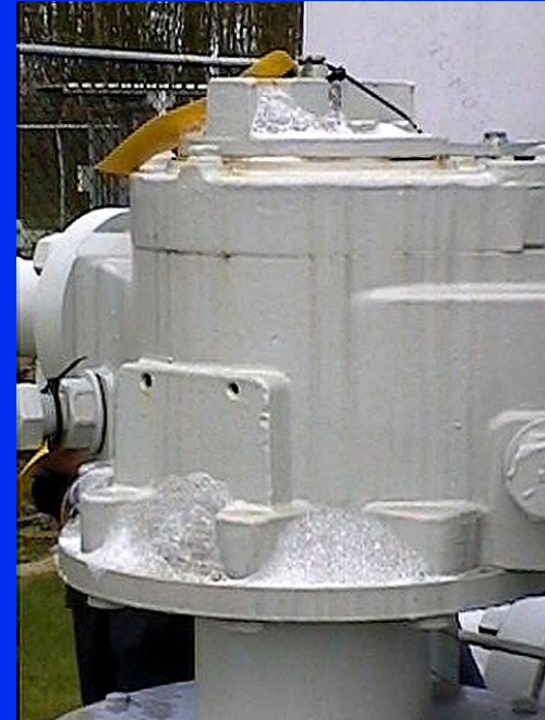
Bubble test on leaking valve
