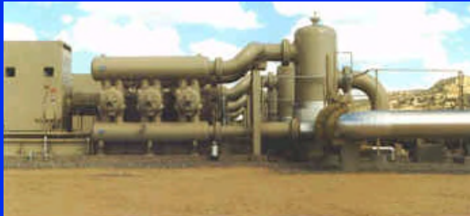
Farmington, New Mexico - Gas Booster Station
