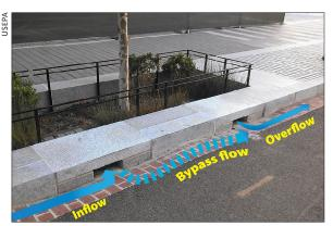
Figure 7. Bypass and overflow system. Runoff enters a planter box through a curb cut and collects until the practice's storage capacity is reached; additional water will either overflow through the second curb cut or will bypass the practice.
