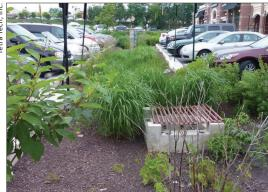
Figure 1. A parking lot bioretention area near Frederick, Maryland, is equipped with an overflow drain.
