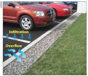
Figure 8. Back up infiltration system. A gravel aggregate strip adjacent to a permeable pavement parking lot collects overflow and directs it into a storm drain or alternative drainage practice.
