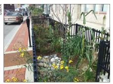
Figure 10. Bioretention planter boxes in Lansing capture and treat much of the stormwater from roads and sidewalks.
