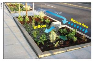
Figure 6. Bypass system. A curb cut allows street runoff to enter this sidewalk planter. If the planter fills completely, additional runoff water volume will be forced to bypass the practice and continue flowing down the road.
