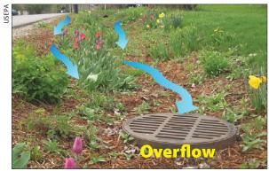
Figure 5. Overflow drain. Runoff water flows into this roadside bioretention channel, which is equipped with an overflow drain to prevent street flooding during high volume storm events.
