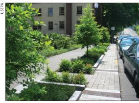
Figure 2. Stormwater planters treat runoff and can bypass flows that exceed their treatment capacity.
