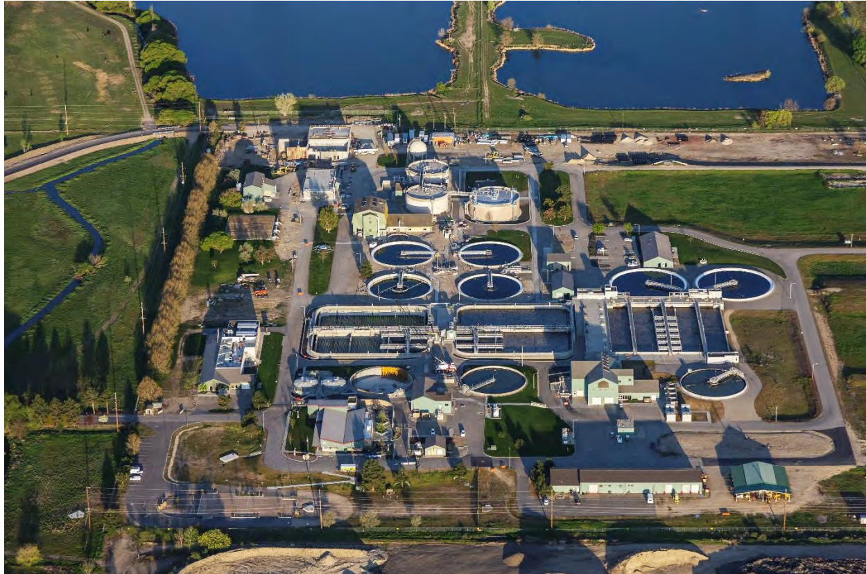
Figure 1. West Boise WWTF – April 2014
