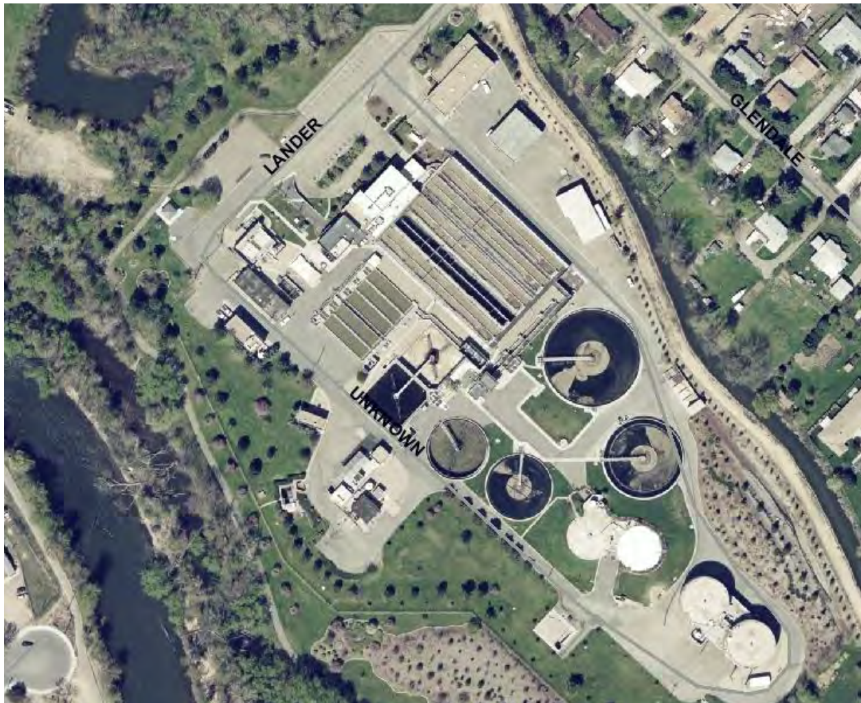
Figure 2. Lander Street WWTF
