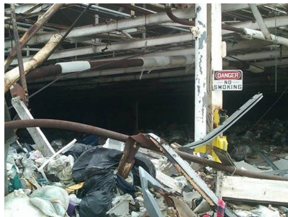
Asbestos TSI on pipes over waste
