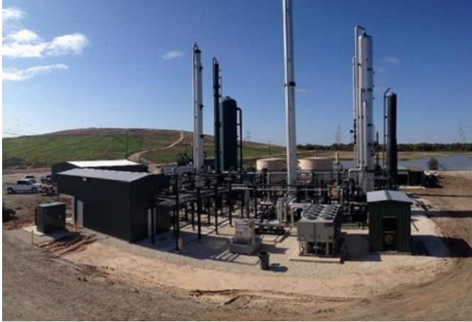
LFG to RNG Plant
