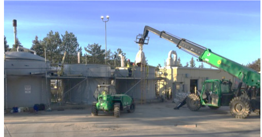
Iron sponge media being loaded into vessels
