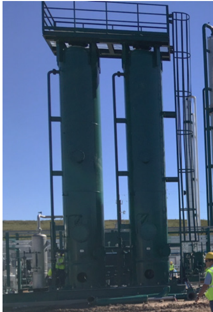
Sulfur removal vessels at a solvent plant
