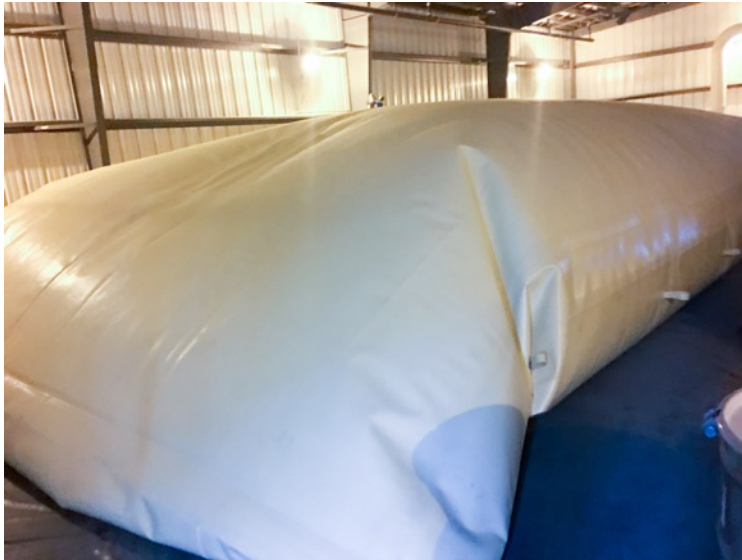
Storage bladder for methane coming off of NRU
