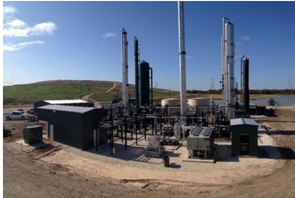
LFG to RNG Plant
