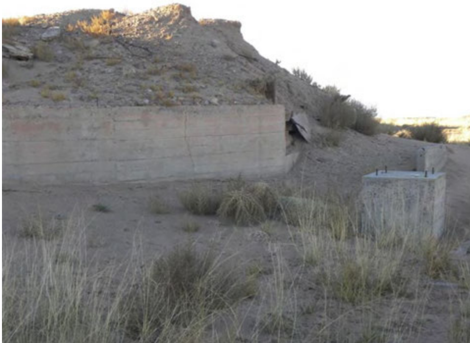
Photo 6. Section 9 Lease, Site #457, concrete structure area
