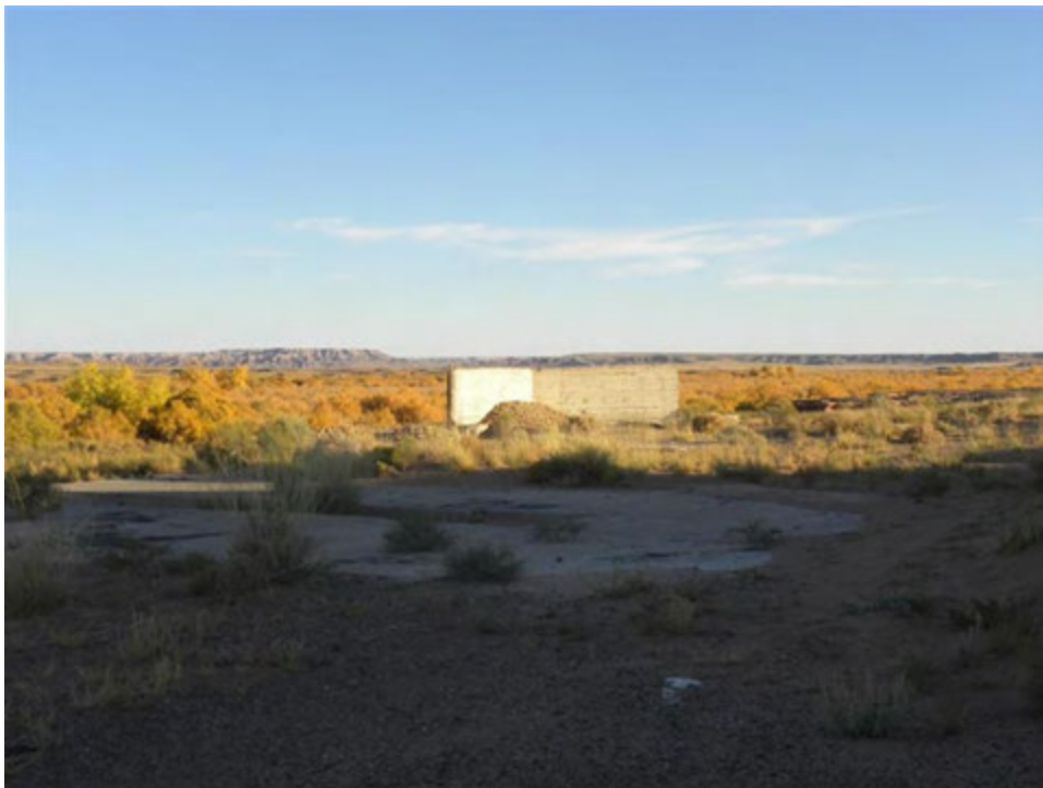
Photo 4. Section 9 Lease, Site #457, concrete structure area
