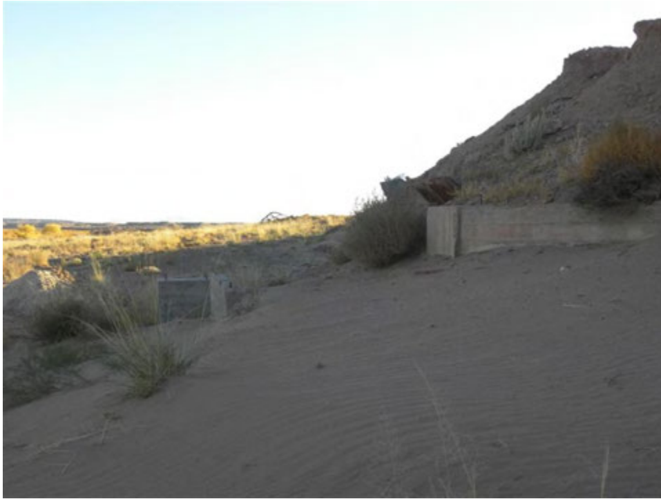
Photo 5. Section 9 Lease, Site #457, concrete structure area
