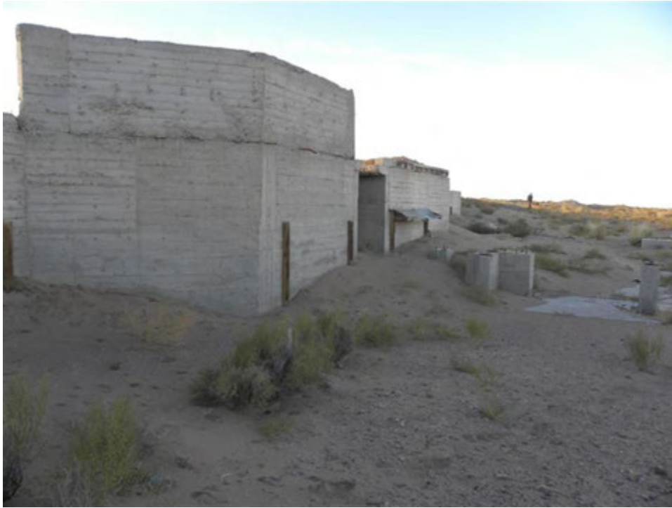
Photo 11. Section 9 Lease, Site #457, concrete structure area
