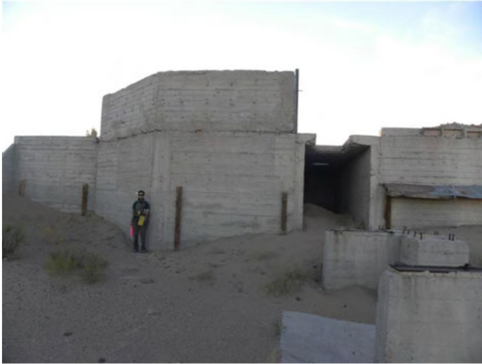
Photo 13. Section 9 Lease, Site #457, concrete structure area
