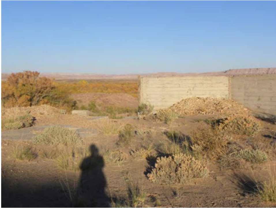
Photo 7. Section 9 Lease, Site #457, concrete structure area
