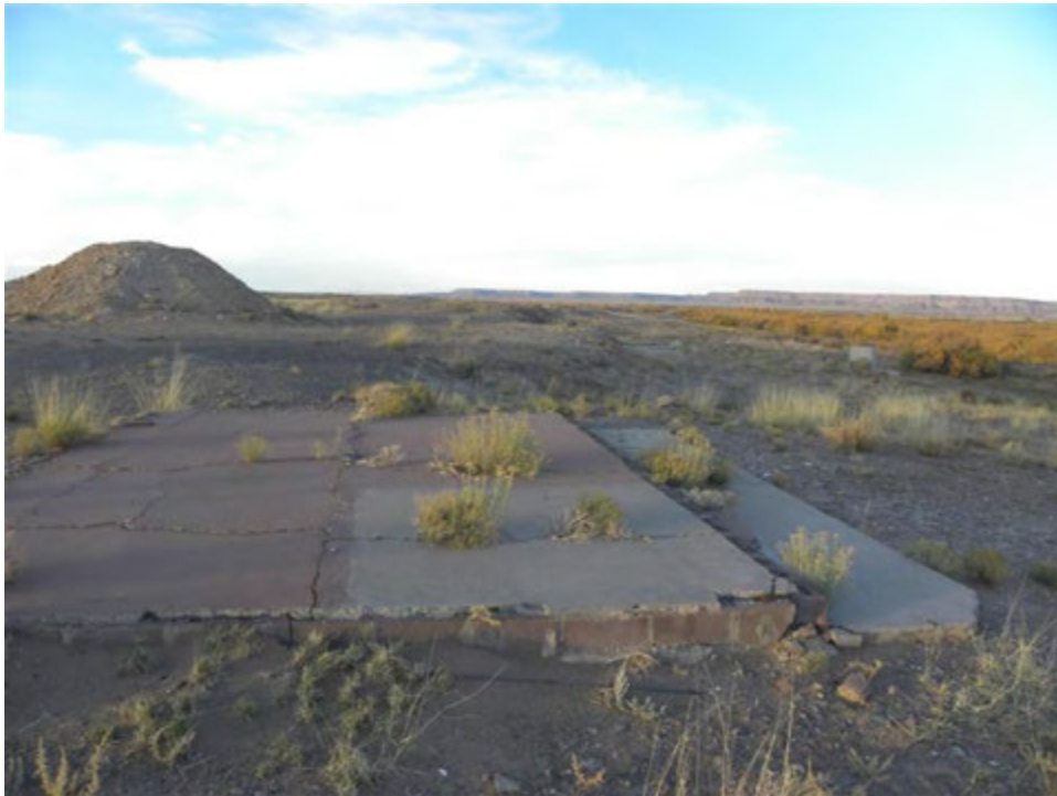
Photo 20. Section 9 Lease, Site #457, foundation south of concrete structure area
