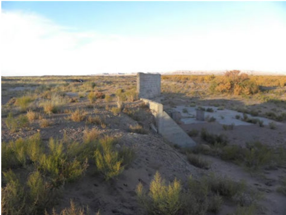
Photo 10. Section 9 Lease, Site #457, concrete structure area
