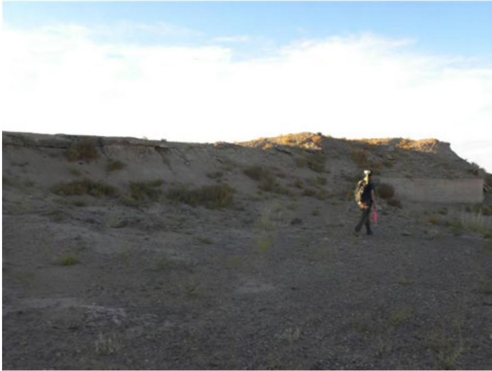
Photo 9. Section 9 Lease, Site #457, concrete structure area
