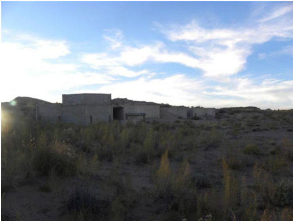
Photo 14. Section 9 Lease, Site #457, concrete structure area
