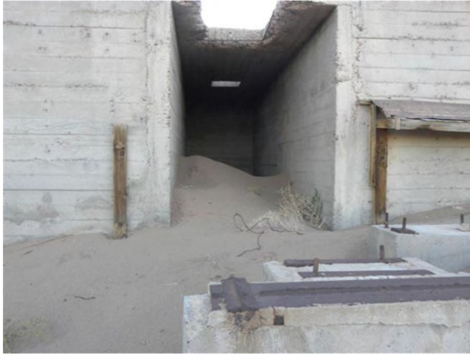
Photo 15. Section 9 Lease, Site #457, concrete structure area
