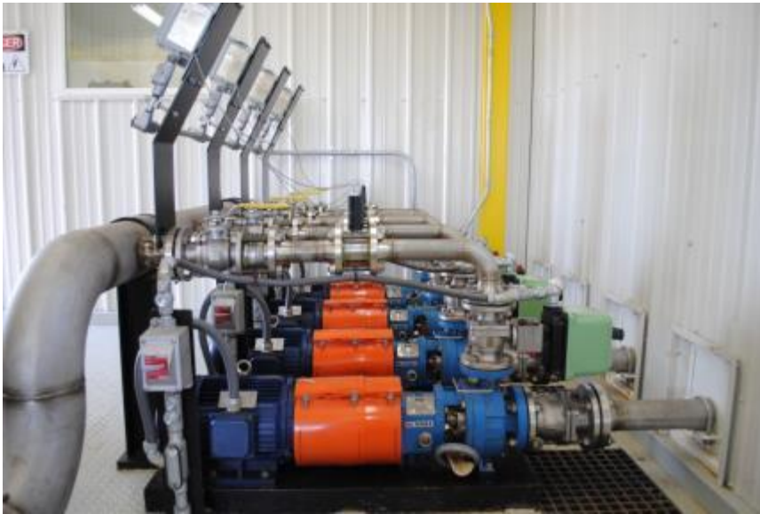
Offload pumps and meters
