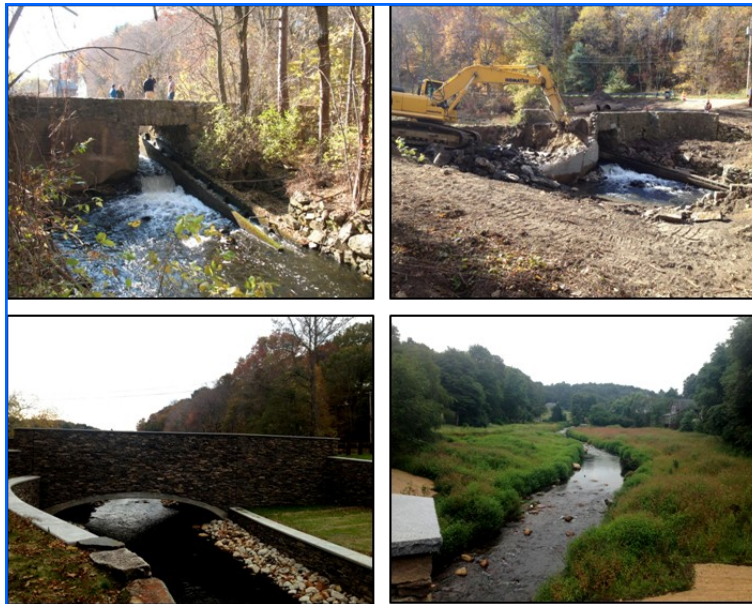
Off Billington Street Dam, Town Brook, Plymouth, removed 2014.
