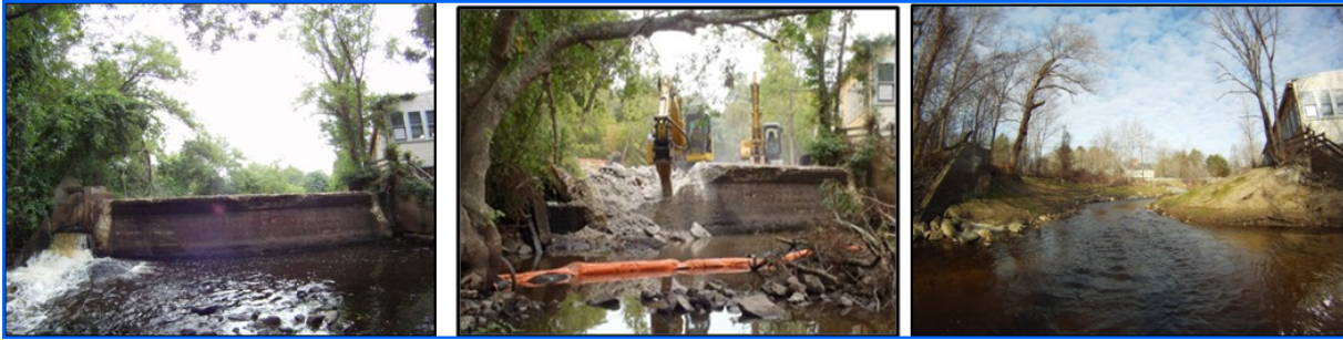
Wapping Road Dam, Jones River, Kingston, removed 2011
