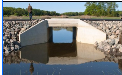
Newman Road Tidal Restoration, Newbury, restored 2010.
