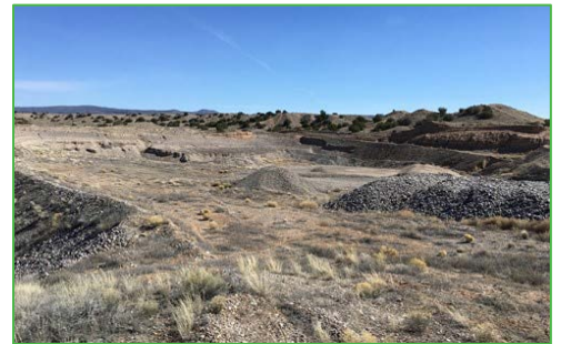
Figure 1. View of the gravel mine site from the southwest corner of the property.
