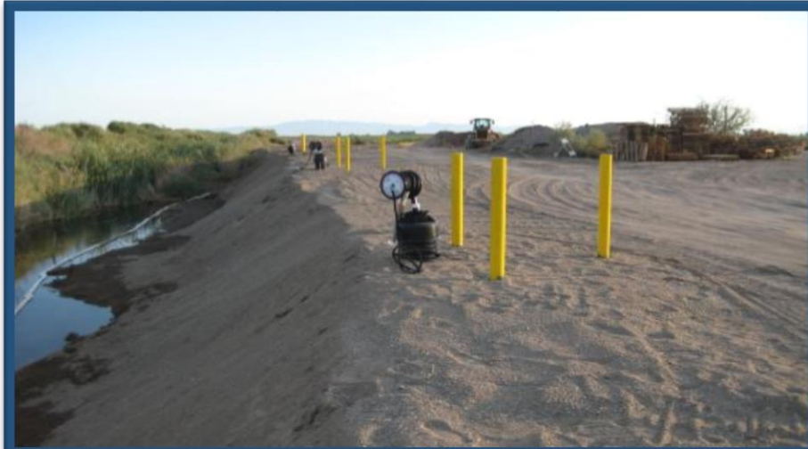
Top of canal bank showing product skimmers used in the remedy at Telles Ranch Photo by Scott Ruth, Bristol Environmental
