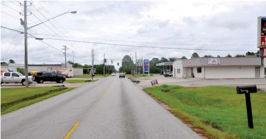
FIGURE 9 An image of the existing street condition along Dedeaux Road looking east.
