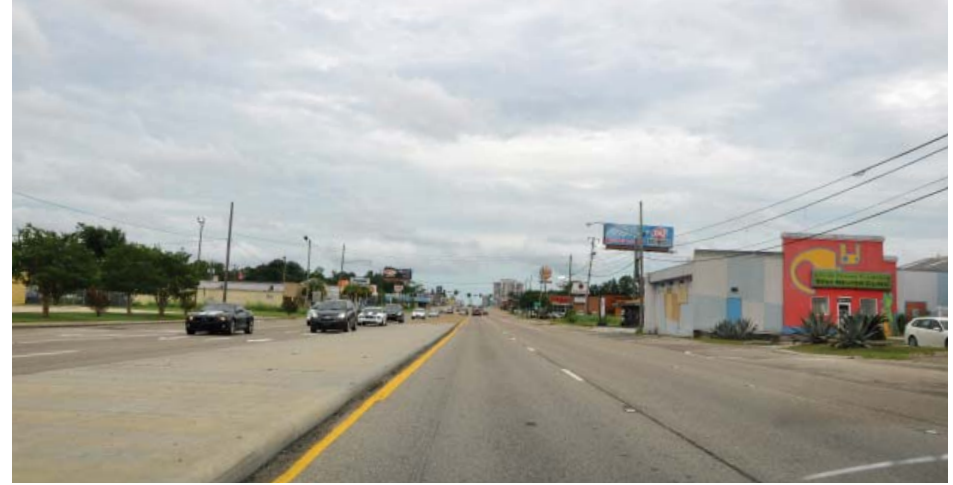
FIGURE 6 An image of the existing street condition along Highway 49 looking south.
