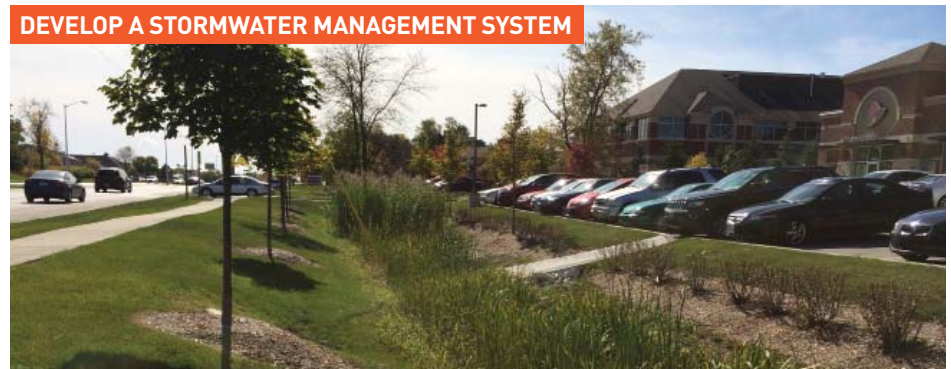
FIGURE 19 The use of a planted grass swale used as a stormwater management system to collect stormwater runoff from roadways and parking lots in new developments of Mequon, Wisconsin. PHOTO CREDIT: Aaron Volkening, flickr.com
