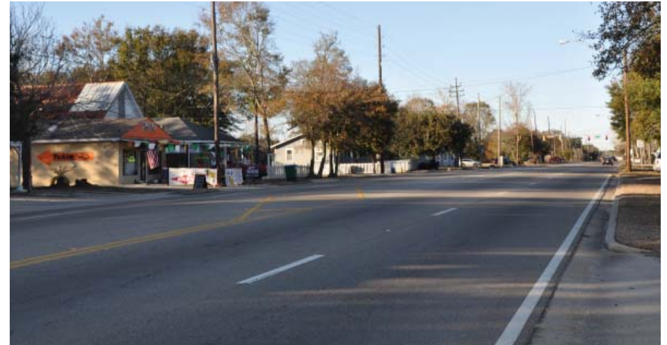
FIGURE 49 An image of the existing street condition along 30th Avenue in the commercial area outside of the Quarters Historic District in the Medical District (east).
