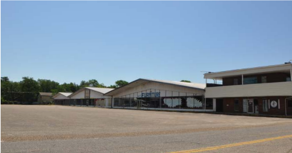
FIGURE 28 An image of a vacant strip mall on Pass Road.
