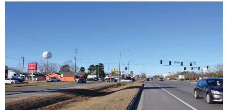
FIGURE 34 An image of the existing street condition along the northern part of Highway 49.
