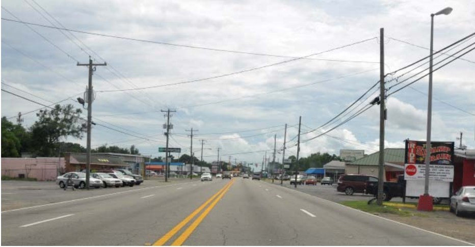
FIGURE 5 An image of the existing street condition along Pass Road looking east.
