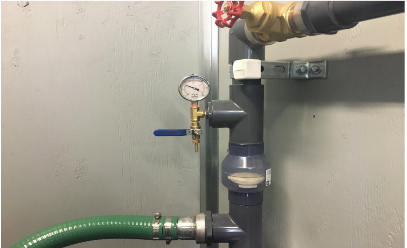
Figure 4 – Outfall 001A/Effluent Sampling Port
