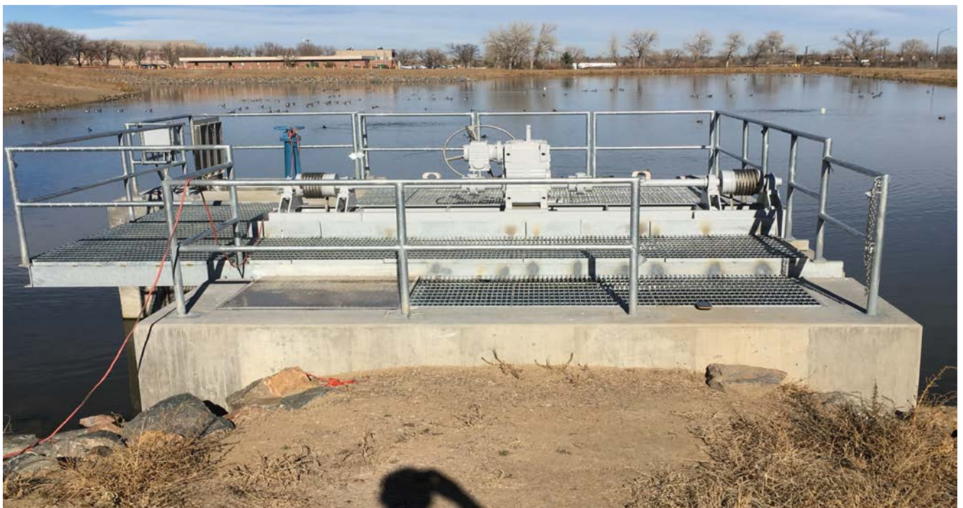
Figure 5 – Downing Reservoir Outlet Structure
