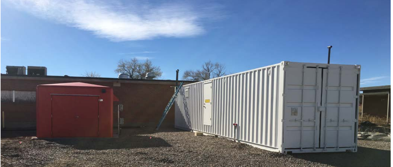
Figure 3 – Downing Reservoir Groundwater Treatment Plant
