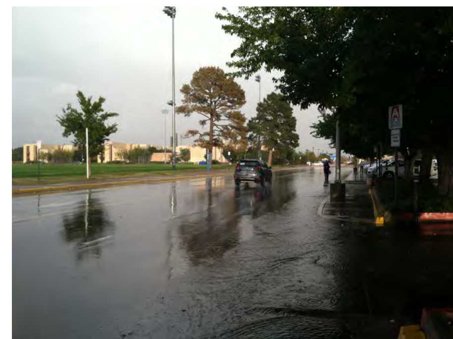
Contaminated and Excessive Run-off South of Field
