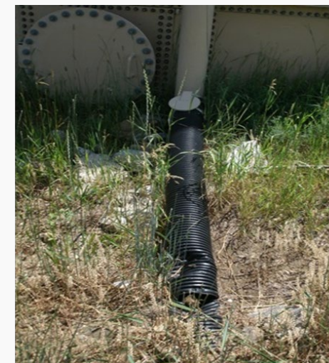
Overflow at ground level (not 12" – 24" above); does not have discharge structure or splashpad
