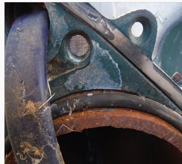
Spider webs in casing showing lack of a sanitary seal
