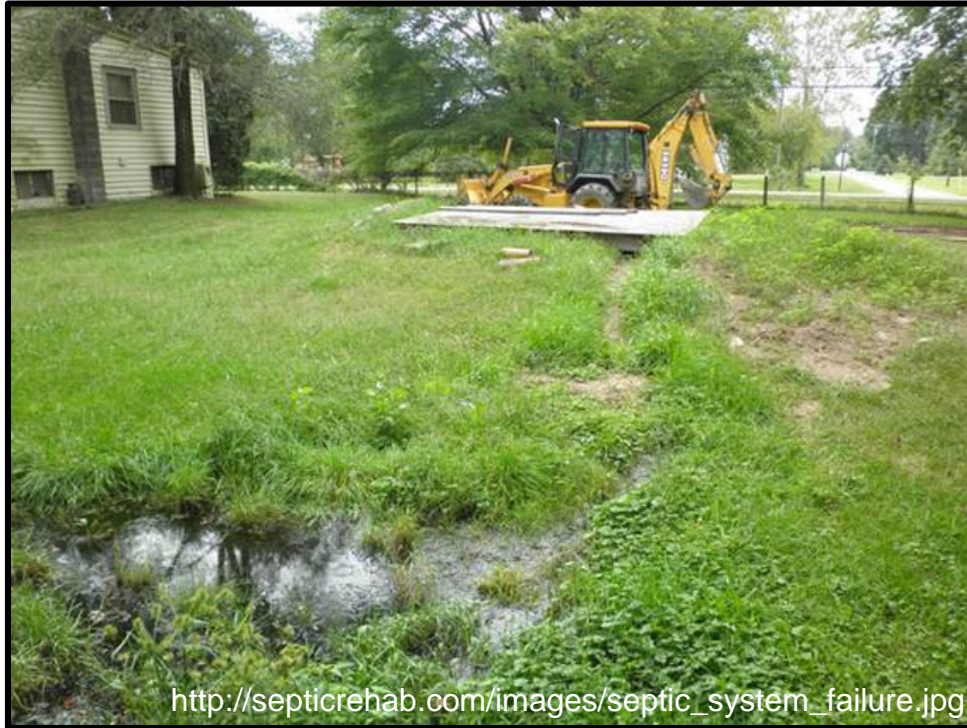
Failing septic system
