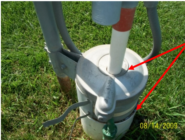
Gaps around pellet chlorinator allowed in irrigated water
