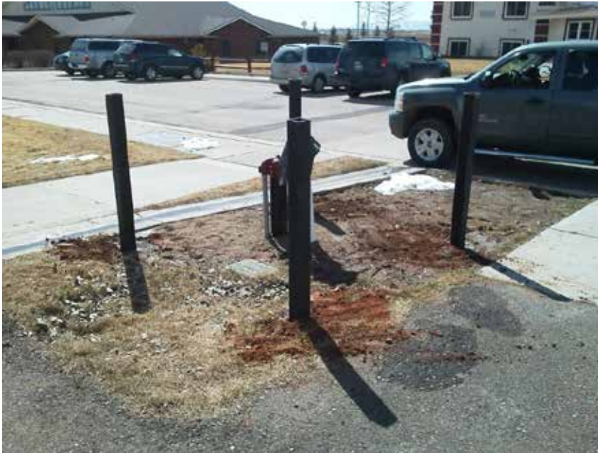
Wells in driveways need to be protected by bollards
