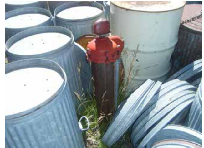
Potential sources of contamination surrounding wellhead
