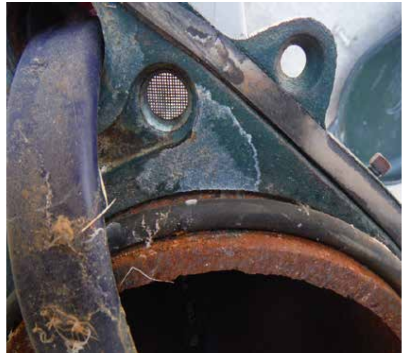
Lack of a sanitary seal
