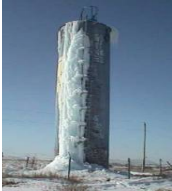
Frozen finished water storage tanks
