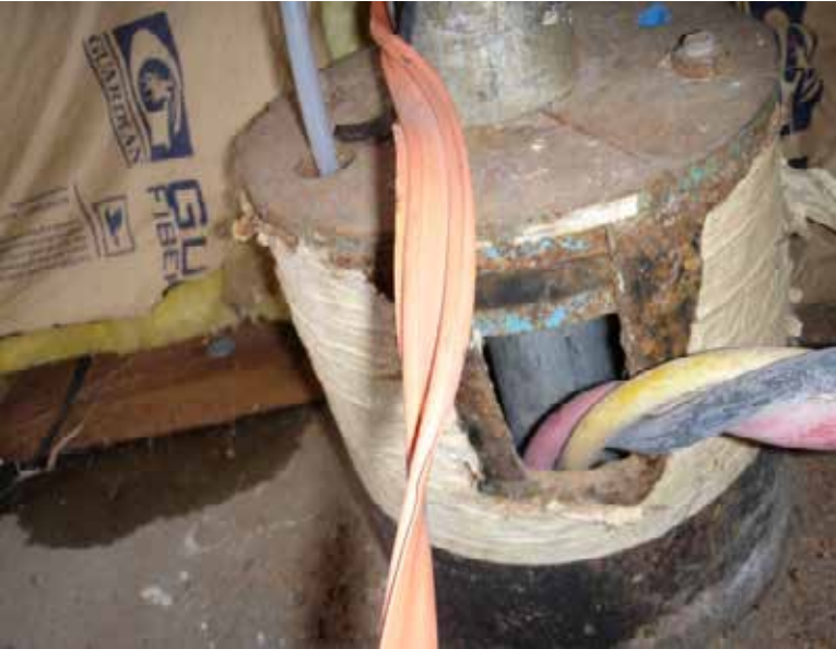
Conduit is not properly sealed.
