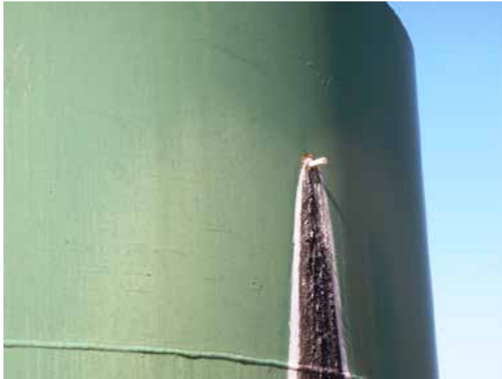
Un-repaired bullet hole in storage tank.
