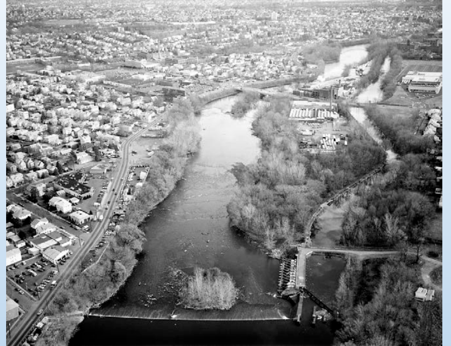
Dundee Dam and Canal, built in 1861. Powered textile factories, later rubber, pharmaceuticals and other chemicals
