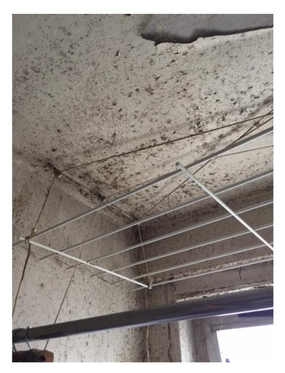
171. Worse, NYCHA has often proven unable to eliminate mold in response to residents' complaints. Although NYCHA eventually cleans the mold from the walls, the mold grows back in many cases because NYCHA does not successfully address its root causes. More than 30% of the time, mold growth returns after NYCHA claims to have addressed it.
