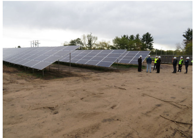
Sky Park Landfill Solar project in Eau Claire, WI.
