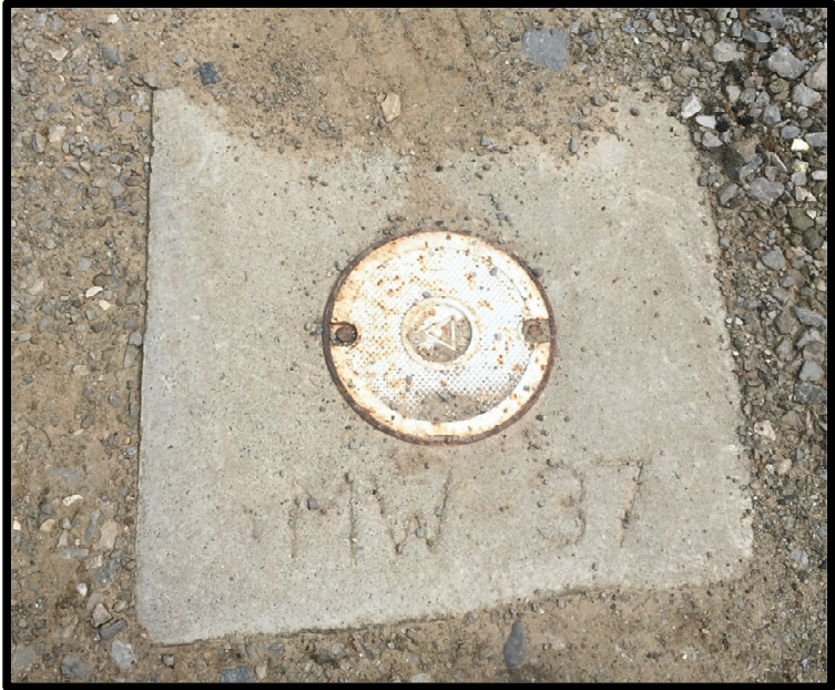
Picture 5: Monitoring Well MW-37
