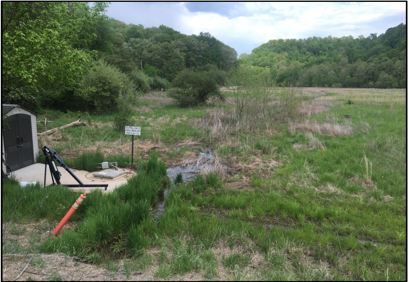
Picture 2: Ward B Landfill and Central Drain Sump Pumping System
