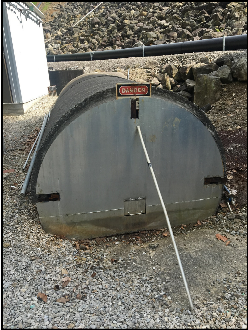
Picture 3: Leachate Collection Tank
