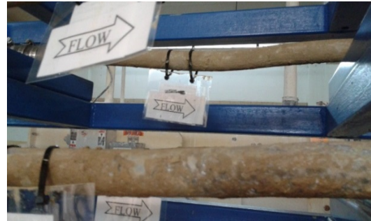
Excavated lead service lines used to test water chemistry at the Flint water treatment plant. (EPA OIG photo)
