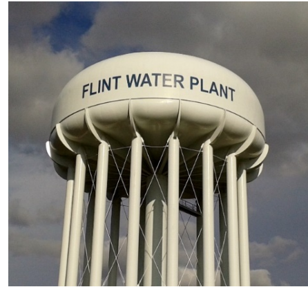
Flint Water Treatment Plant. (EPA OIG photo, taken April 2016)
