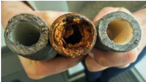
Lead service lines showing inner surface without any coating from corrosion control treatment (left), with coating (right), and fully corroded (middle). (EPA photo)
