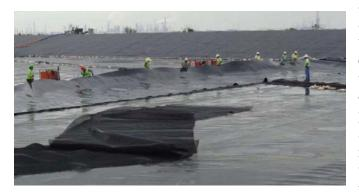
Liner being installed in base of RCRA cell at the Malone Service Company hazardous waste cleanup site, Texas. (EPA photo)
