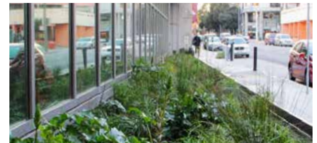
Figure 44. The constructed wetland technology is coined "The Living Machine." The wetlands are in raised planters located between the sidewalk and building. Image source: Biohabitats, Inc.
