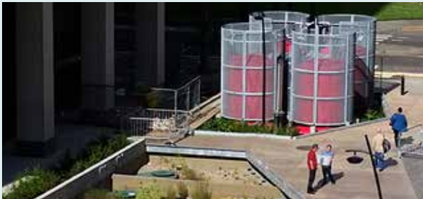
Figure 42. Hassalo on 8th has an onsite wastewater treatment system coined "NORM" (Natural Organic Recycling Machine). The components include both trickling filters (red towers) and constructed wetland technologies to meet water quality suitable for reuse as irrigation, toilets, and makeup water for cooling. Image source: Biohabitats, Inc.
