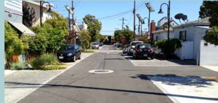
Figure 8. Longfellow Street in Santa Monica, CA is curbless and has no sidewalks. The entire street can be shared by all users. Permeable pavers and landscape planters define parking areas and visually narrow the drive aisle. Cross street intersections are depressed, continuing the curbless street and paver treatments for a uniform appearance and function. Image source: Sherwood Design Engineers
