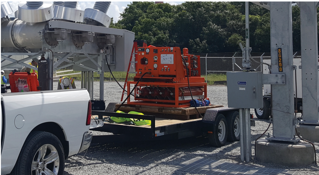
Figure 7. A gas cart can enable employees to more efficiently handle SF 6 .
