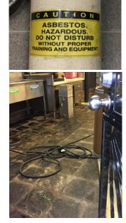
Top: Asbestos warning label on piping in a school's boiler room. Bottom: Floor tile replacement in a school kitchen. (EPA OIG photos)
