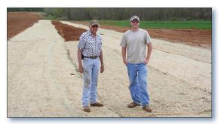
Figure 2. Erosion control blankets were used to stabilize eroded cropland, preventing sediment and nutrients from washing into the creek.
