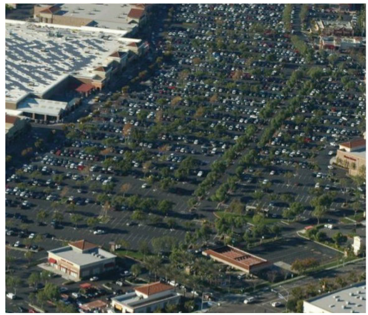
Shading from trees, buildings, cars etc. may lessen urban heat island reduction potential of pavements
