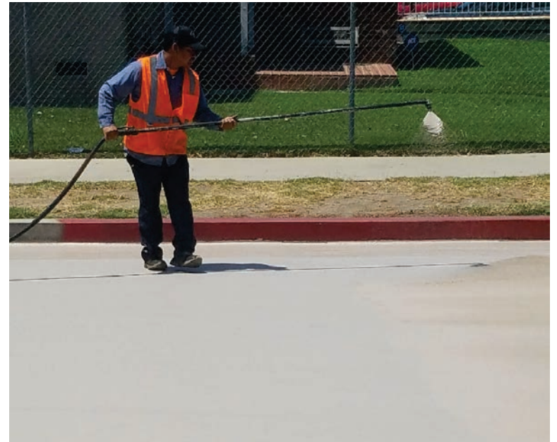
Second coat applied by hand spray
