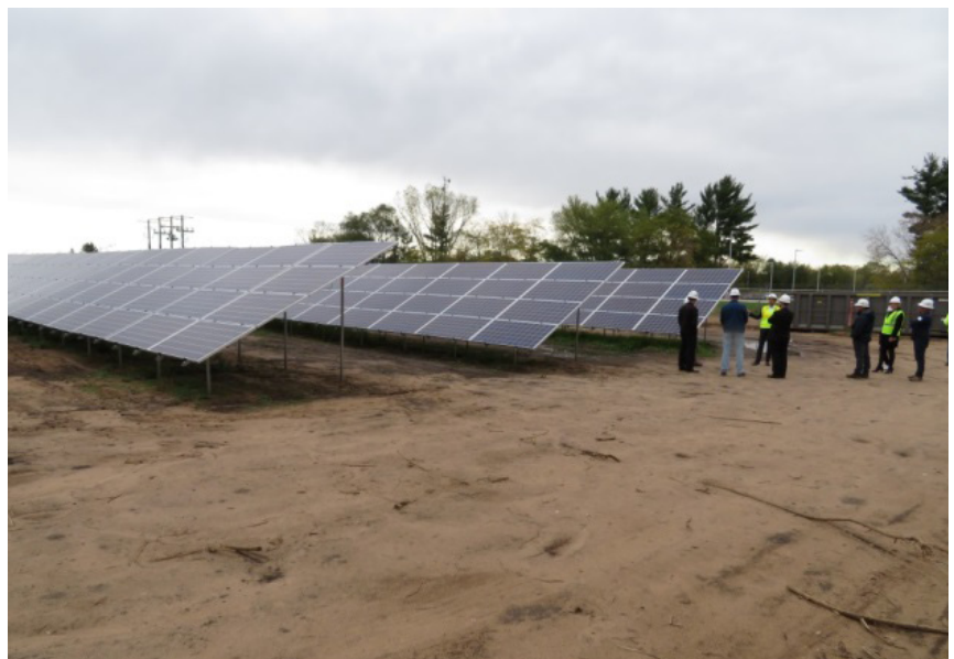
Sky Park Landfill Solar. Photo Credit: City of Eau Claire
