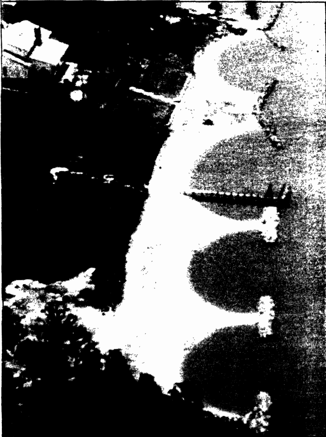
Figure 6-17. Headland breakwater system at Drummonds Field, Virginia. The breakwaters control shoreline erosion and provide a community beach. (Hardaway and Gunn, 1991.)
