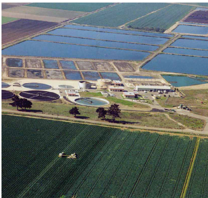
Aerial view of the Santa Maria WWTP.
