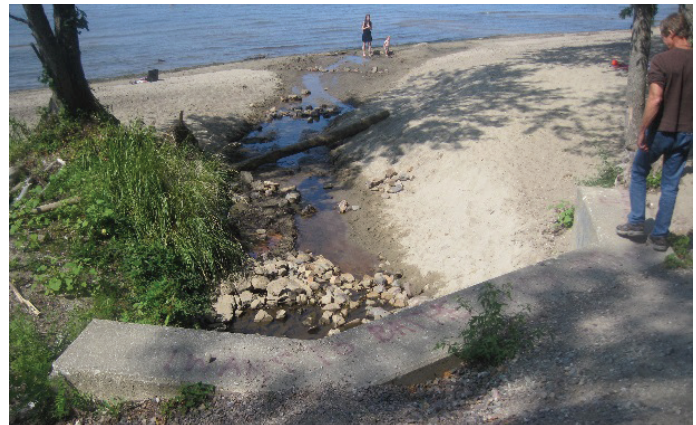
Stormwater outfall near a popular recreational beach on Lake Champlain in Burlington. Barry Tanning, Tetra Tech
