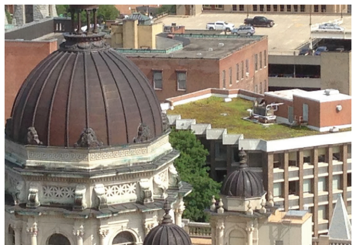
Green roof in the combined sewer area of downtown Syracuse. A wide range of stormwater projects in this area have reduced CSO overflow events and volumes in recent years. Barry Tanning, Tetra Tech
