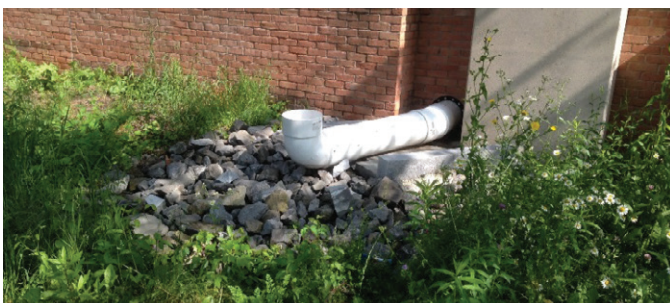
Downspout disconnection and flow dispersal for infiltration in Syracuse help reduce stormwater volumes that exacerbate CSOs and contribute to “flashy” runoff episodes. Barry Topping, Tetra Tech
