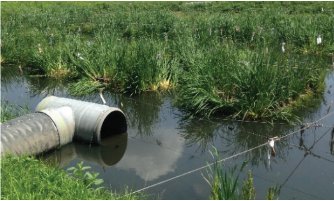
Large stormwater treatment wetland installed by the “Save the Rain” program near Onondaga Lake. Barry Tanning, Tetra Tech
