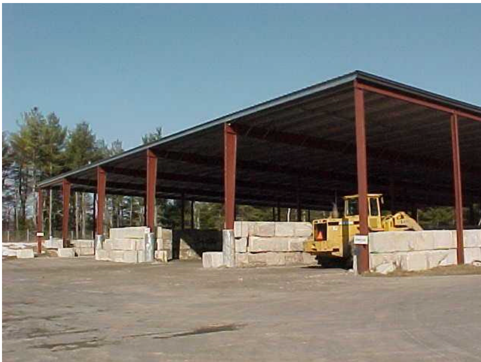
Figure 5-5. Permanent covered storage in Southern Maine (Courtesy Mark King, Maine Dept. Environmental Protection).
