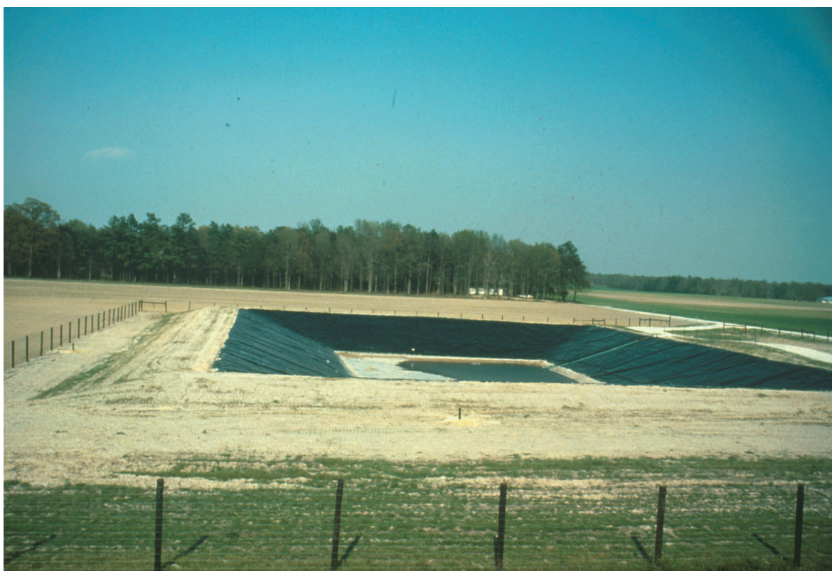
Fig. 5-5 A lined lagoon (Courtesy of BioGro Division).
