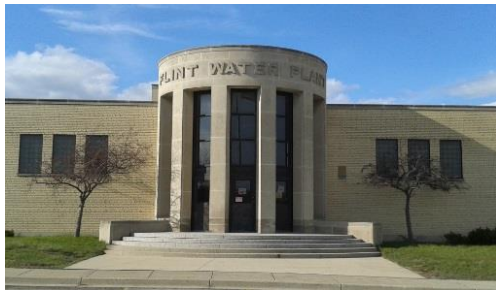
Flint Water Plant, Flint, Michigan. (EPA OIG photo)
