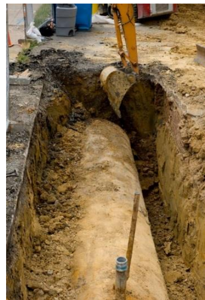
An underground storage tank being removed. (EPA photo)
