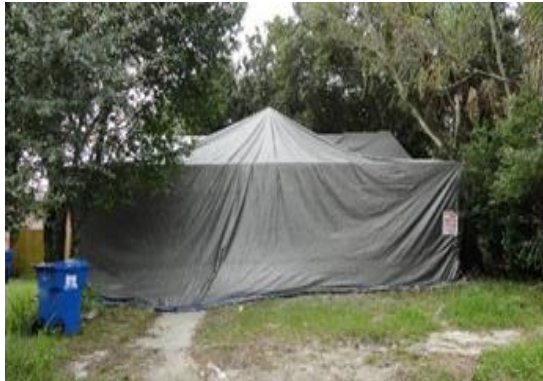
A Florida residence is fumigated with sulfuryl fluoride to combat drywood termites. (EPA photo)
