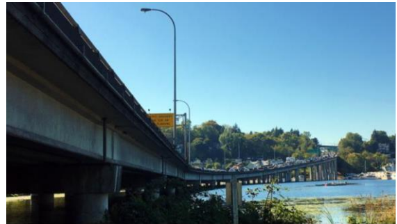
SR-520 bridge traffic in Seattle. Drain pipes visible at each column allow contaminated stormwater to flow directly from the roadway into Portage Bay, Union Bay, and Lake Washington.
