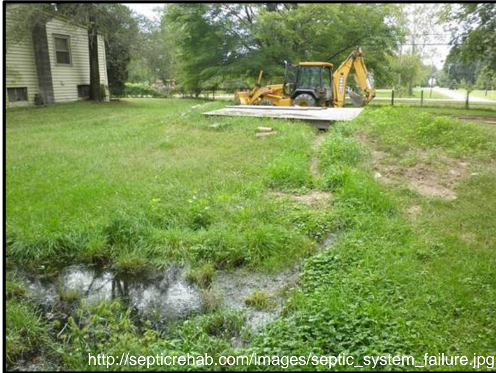
Failing septic system
