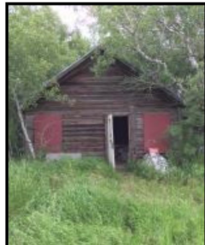
Preserved Historic Dance Hall Building
