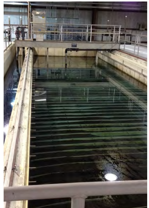
Views of the capped pond area and groundwater treatment facilities at the Milan Army Ammunition Plant site.
