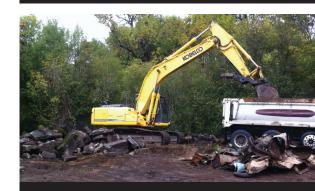
Workers removed concrete rubble and hazardous containers from the property and remediated groundwater contamination.
