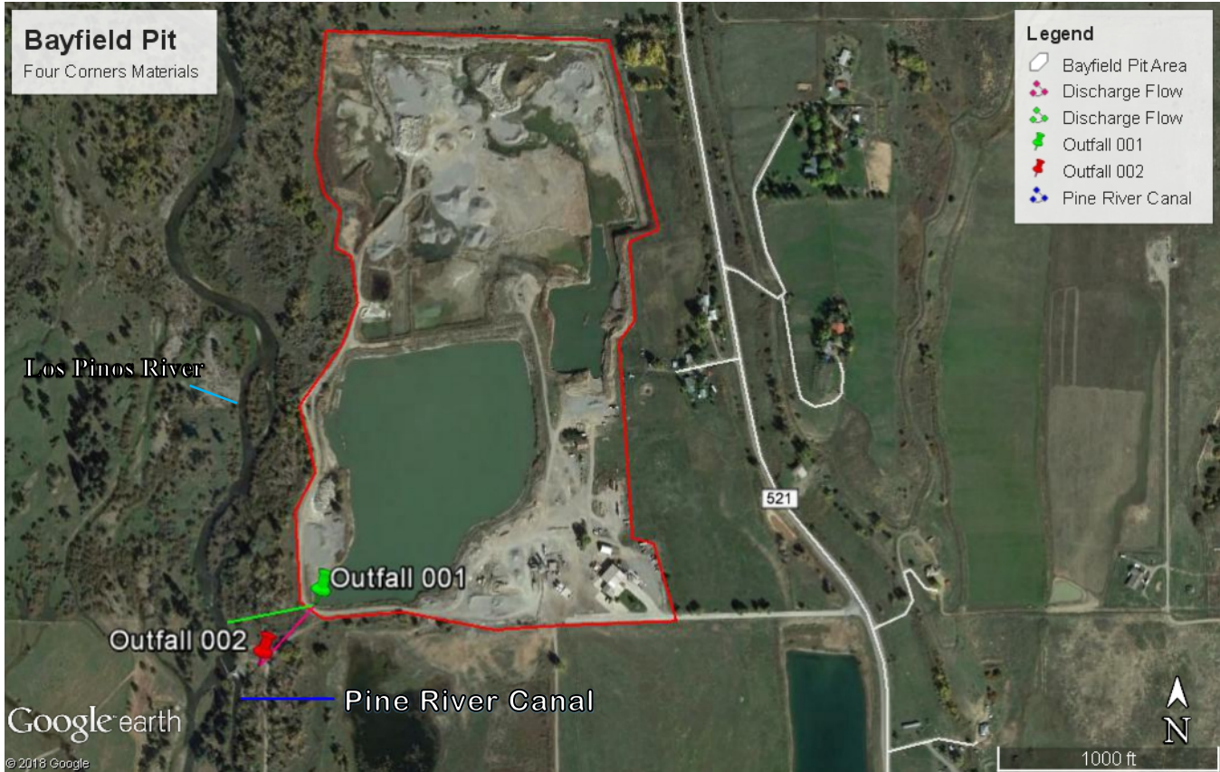
Figure 1. Facility Aerial Map
