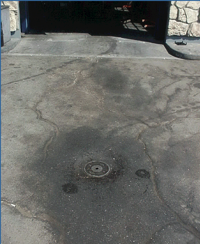
Closeup of manhole to seepage pit
