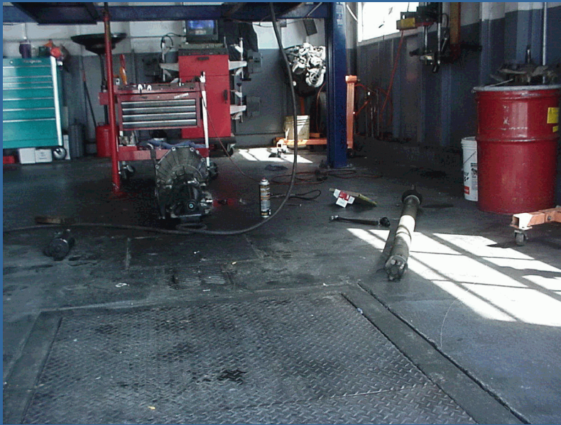
Repair bay with drain and clarifier cover
