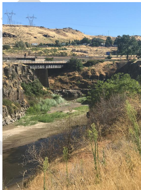
Photo 7-58 Looking upstream from the confluence toward the Fifteenmile Creek flow
