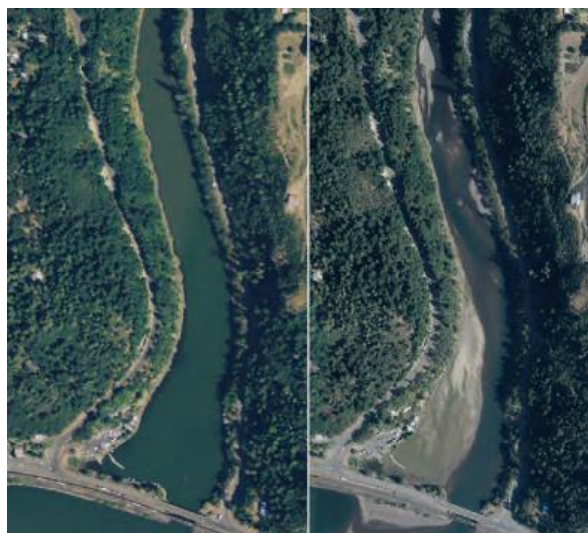
Photo 7-44 White Salmon River confluence before and after the removal of the Condit Dam; USGS, U.S. Department of Interior, 2015
