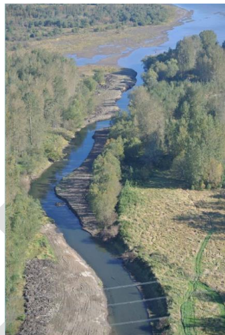
Photo 7-15 East Channel post-Sandy Delta Diversion Dam removal (USACE)
