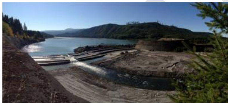
Photo 7-5 Sediment retaining structure on the north fork of the Toutle River, which eventually flows to the Cowlitz
