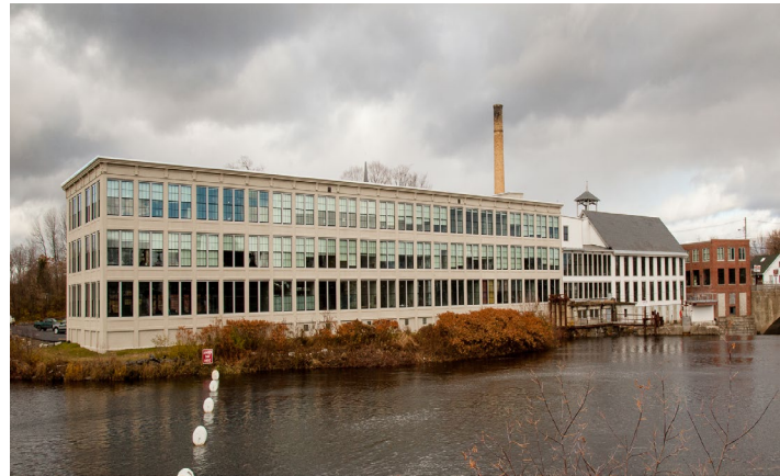
Mayo Mill Redevelopment
