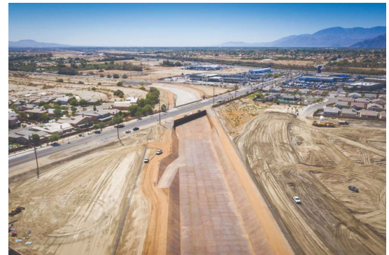
North Indio Regional Flood Control Project Photo Credit: Coachella Valley Water District
