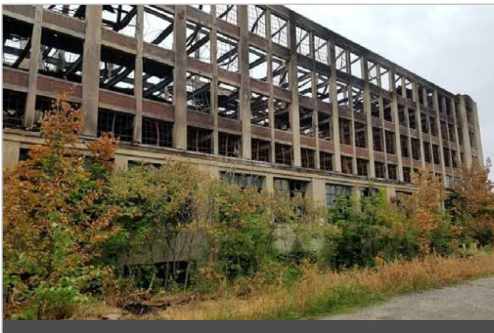
Stenton Trust Mill Building
