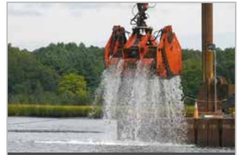
Dredging of New Bedford Harbor
